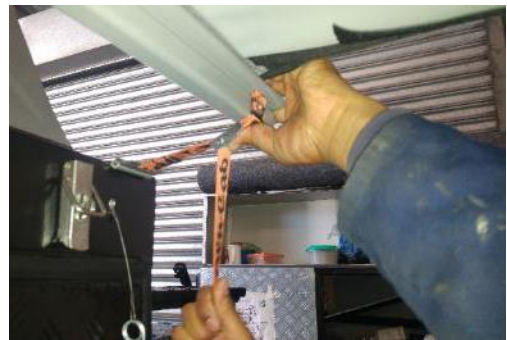
Figure 14: Tightening of strap
