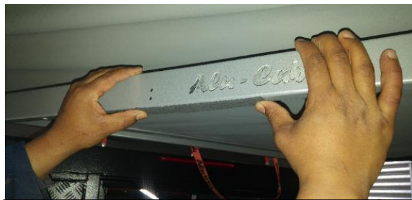
Figure 16: Black Adhesive foam strip attached
